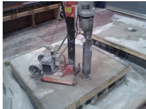
(b) Drilling process
