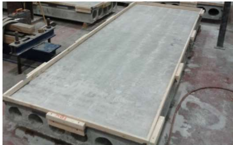
(a) Before casting the topping
