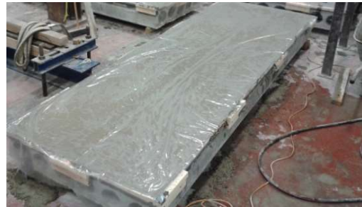
(b) After casting the topping
