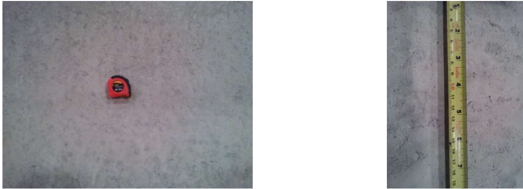
Fig. 1: Surface finish of slab MA1
