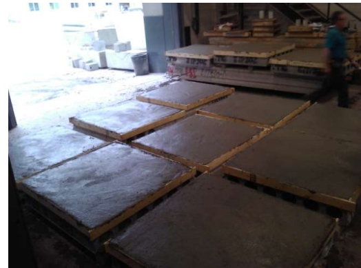
(b) After casting the topping
