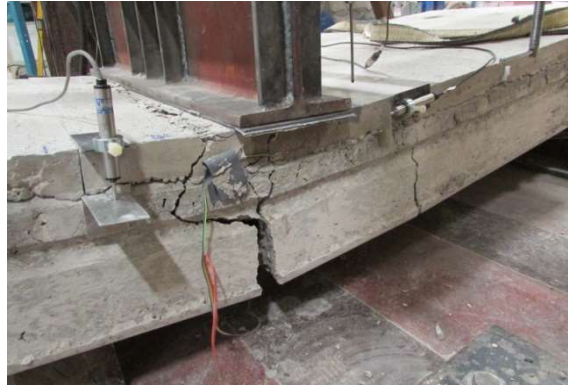
Fig. 23: Slab at failure
